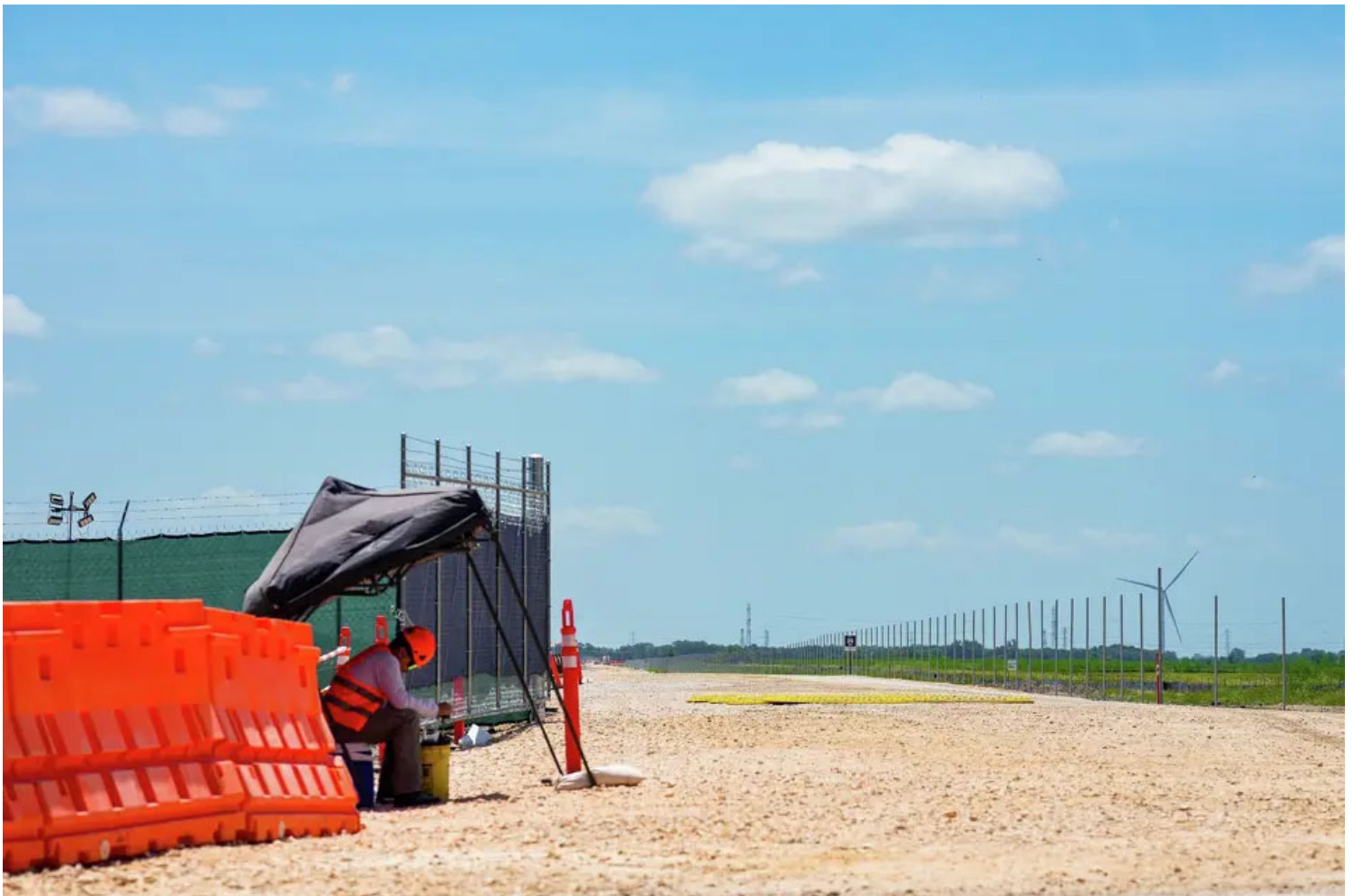
The entrance to Amazon's data center construction near Boling photographed on July 31, 2026. Raquel Natalicchio/Houston Chronicle
