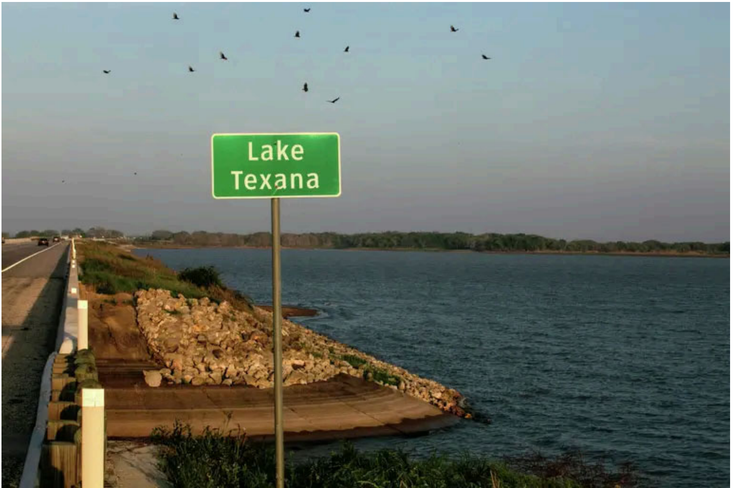
Corpus Christi's largest remaining reservoir, Lake Texana, is currently 55% full and projected to hit 30% this summer. Dylan Baddour/Inside Climate News
