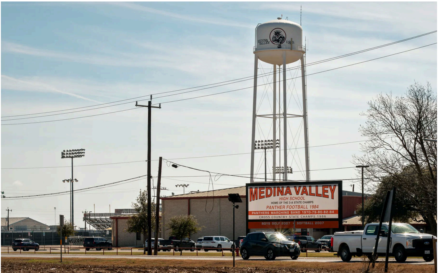
A water tower in Medina County. Reid Bader
