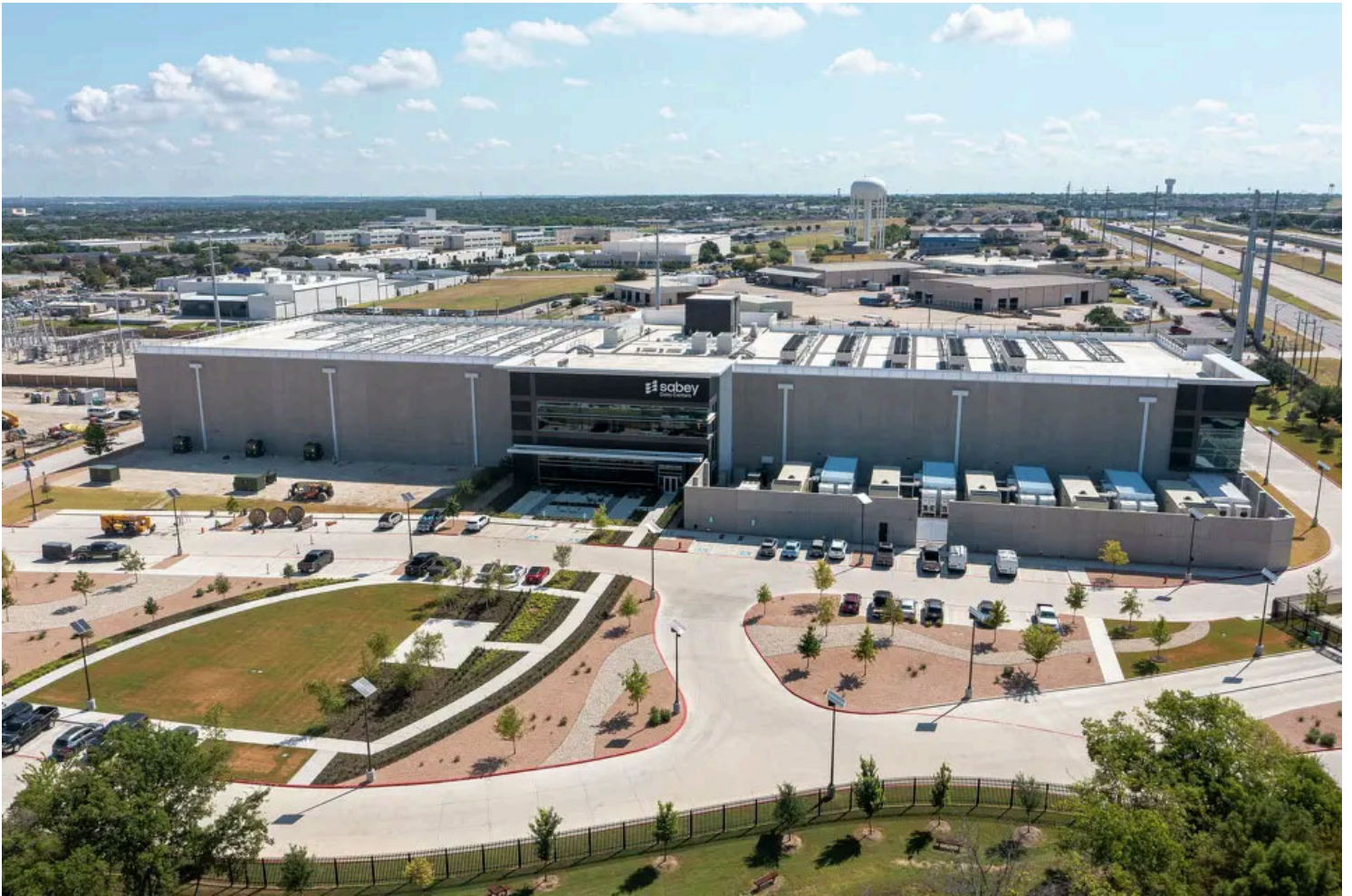
The Sabey Data Center in Round Rock, Texas on Monday, Aug. 11, 2025. Aaron E. Martinez/Austin American-Statesman
