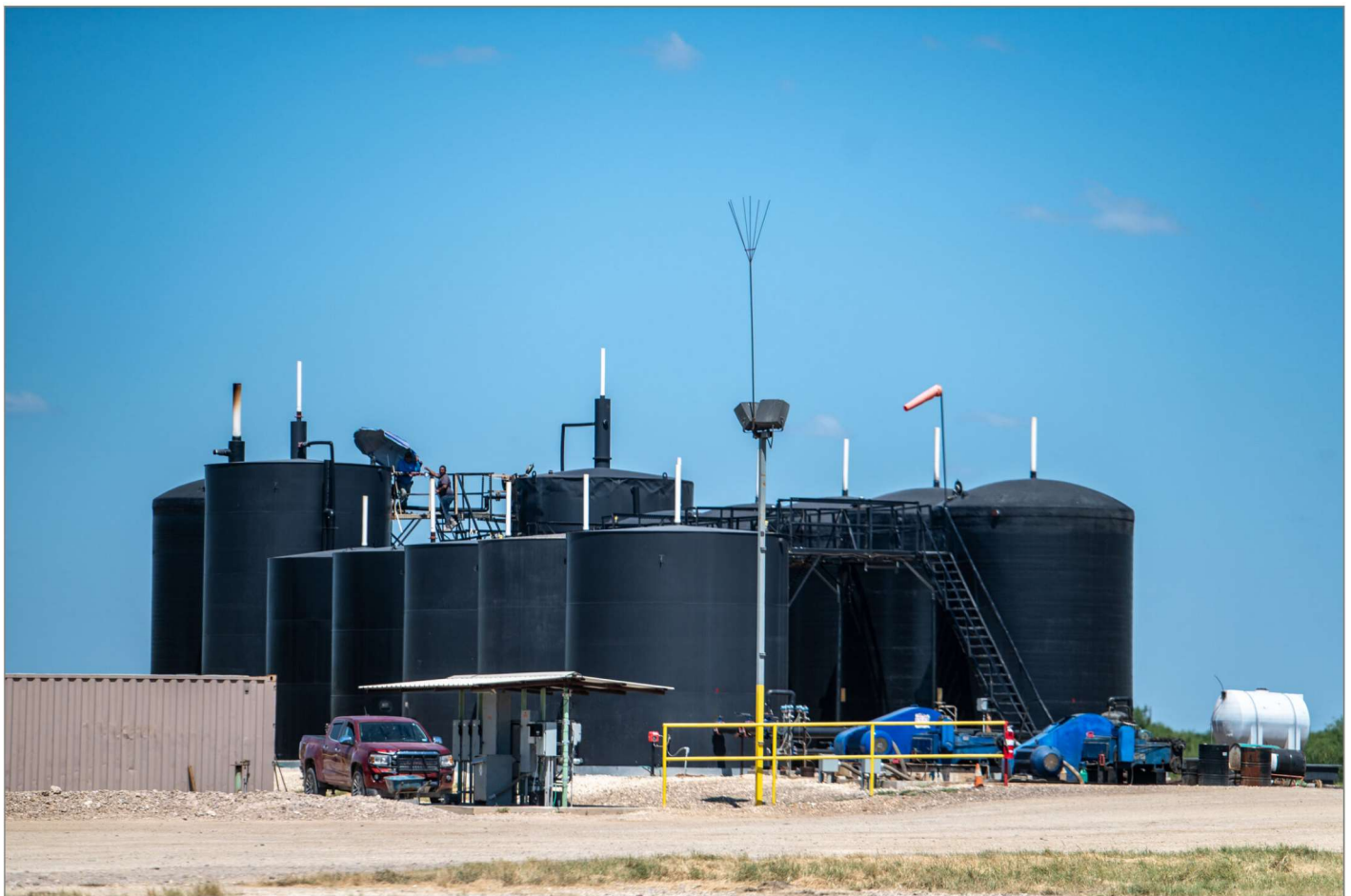
Fracking wastewater tanks near Big Wells, Texas. Sergio Flores for The New York Times
