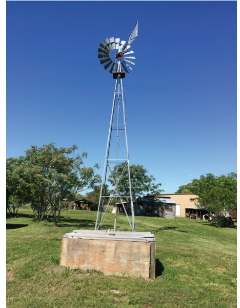
Duncan Windmill: Windmill pumps from a 600-foot deep well into a large concrete cistern that was dug by hand.
