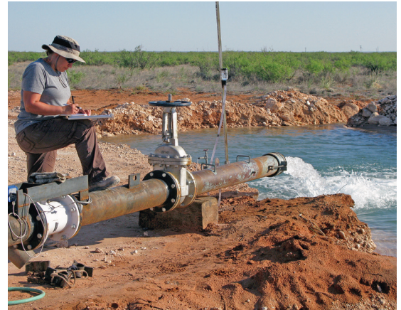
Monitoring a pumping test of a completed production well
